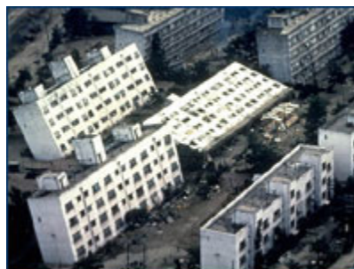
Damage due to liquefaction after an earthquake in Niigata, Japan in 1964.
